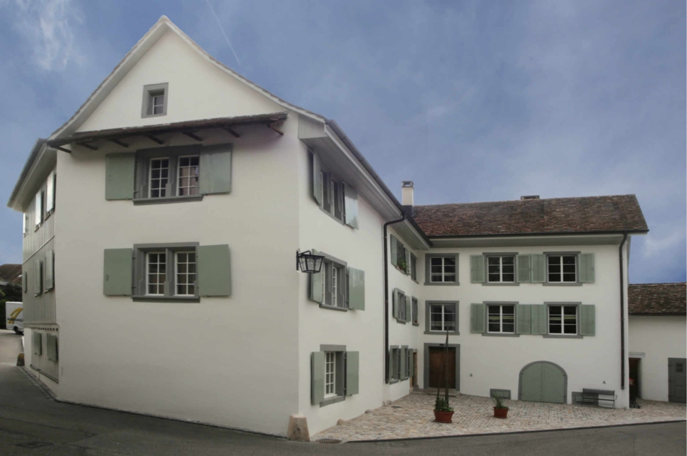
Apartment building 'Alte Mühle' renovation Sissach
