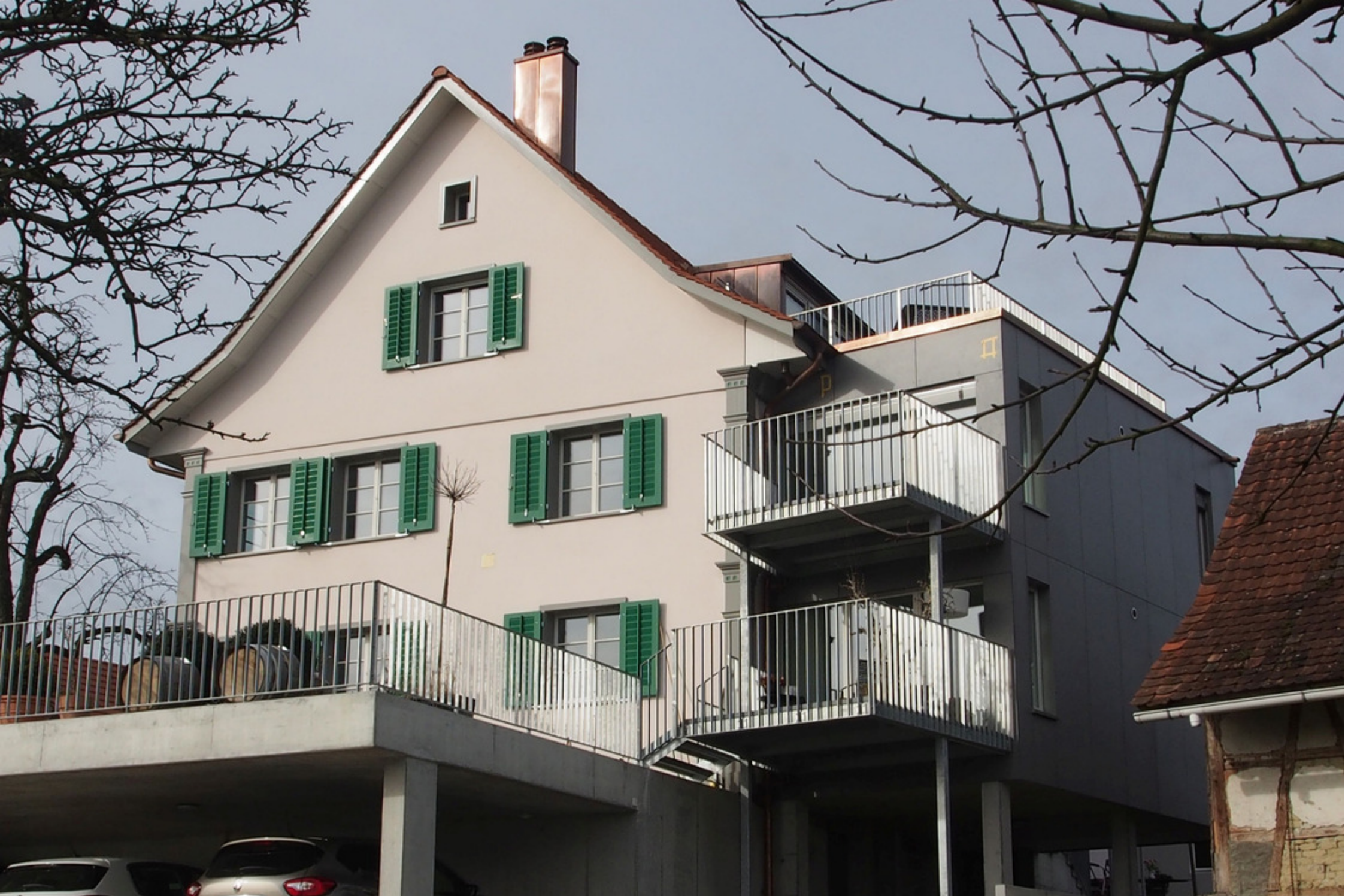
Multi-family house renovation Steinebrunn
