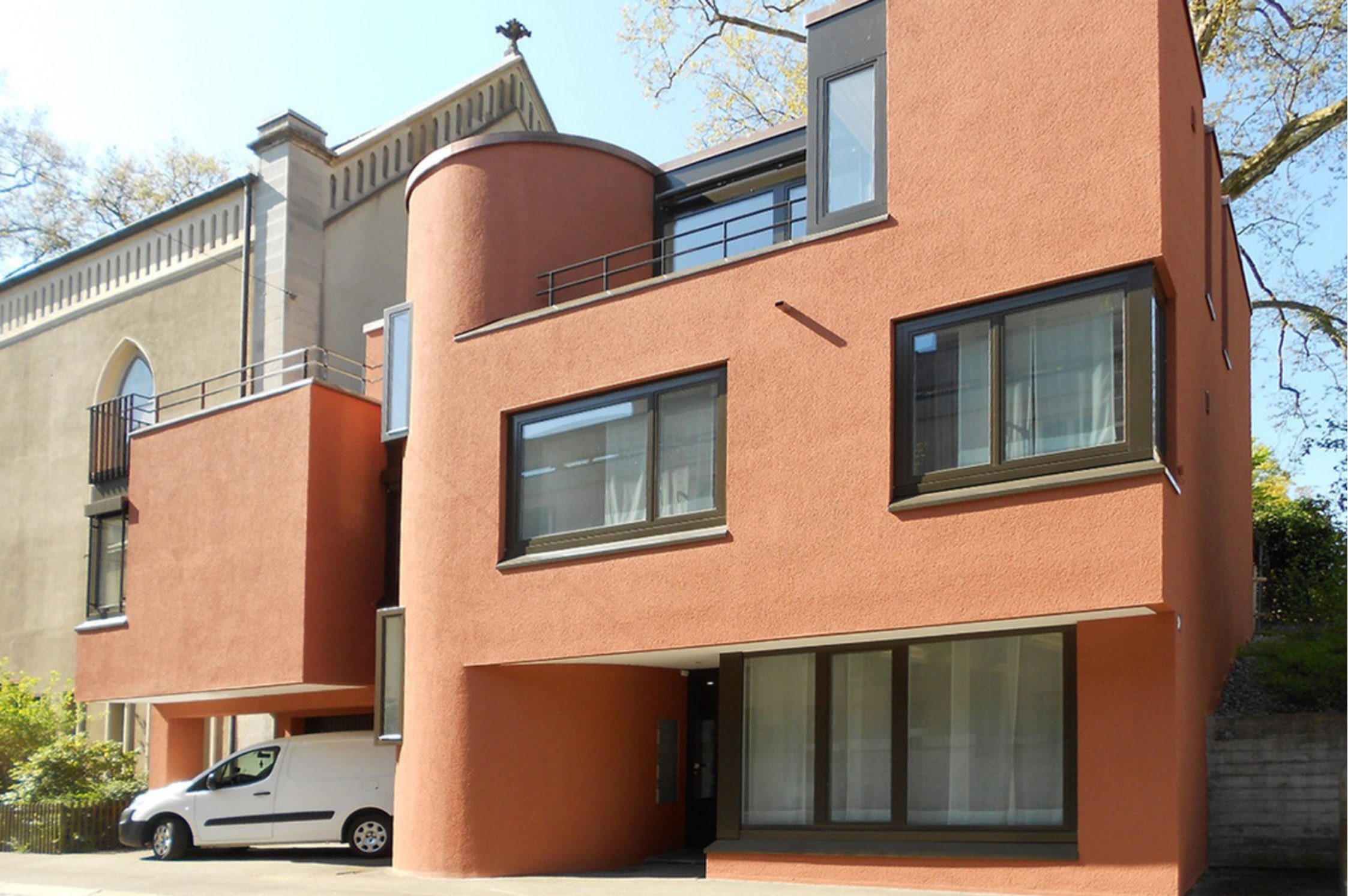
Modern church renovation in Zurich
