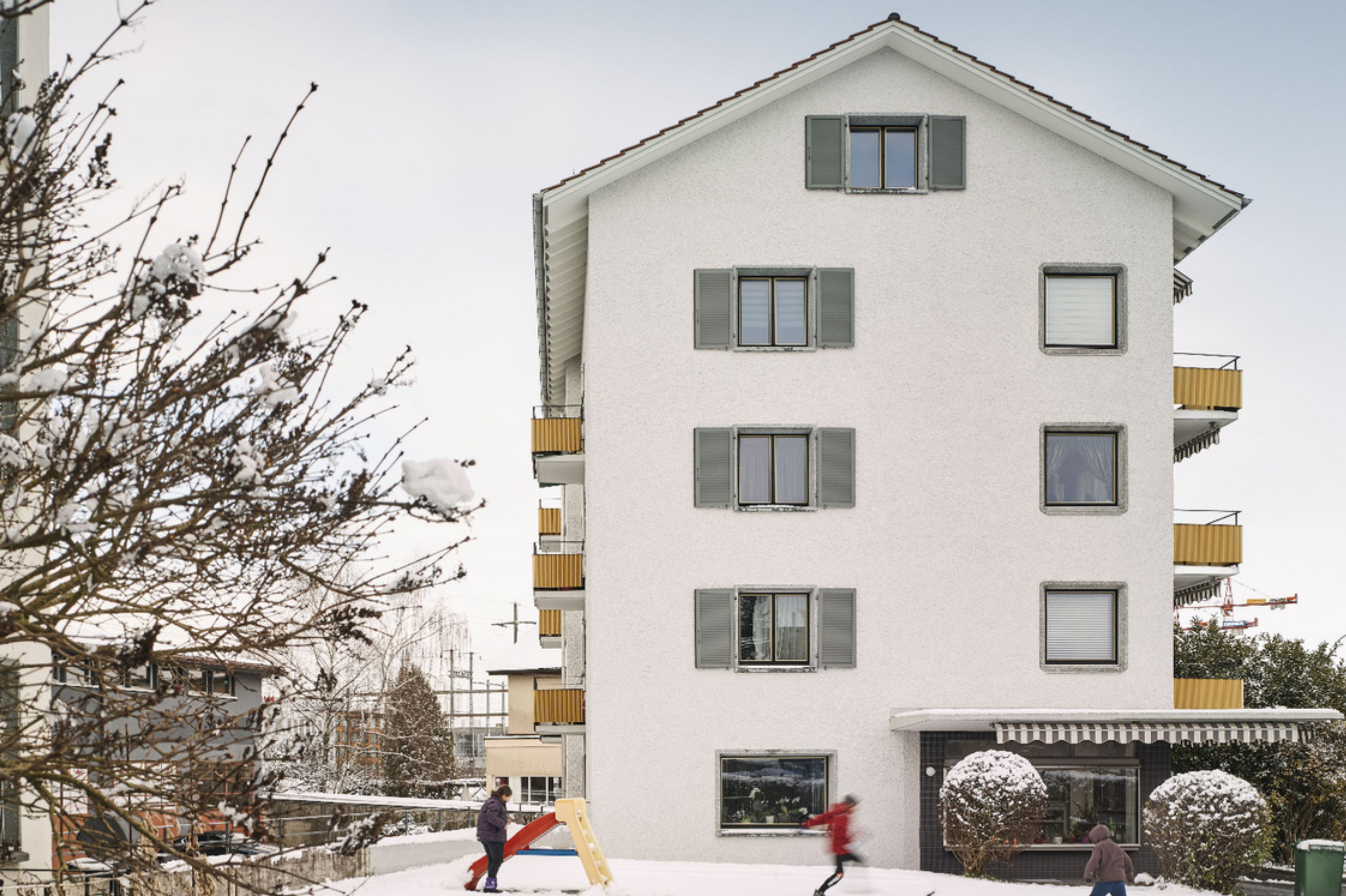
Apartment building Ifangstrasse renovation Rümlang
