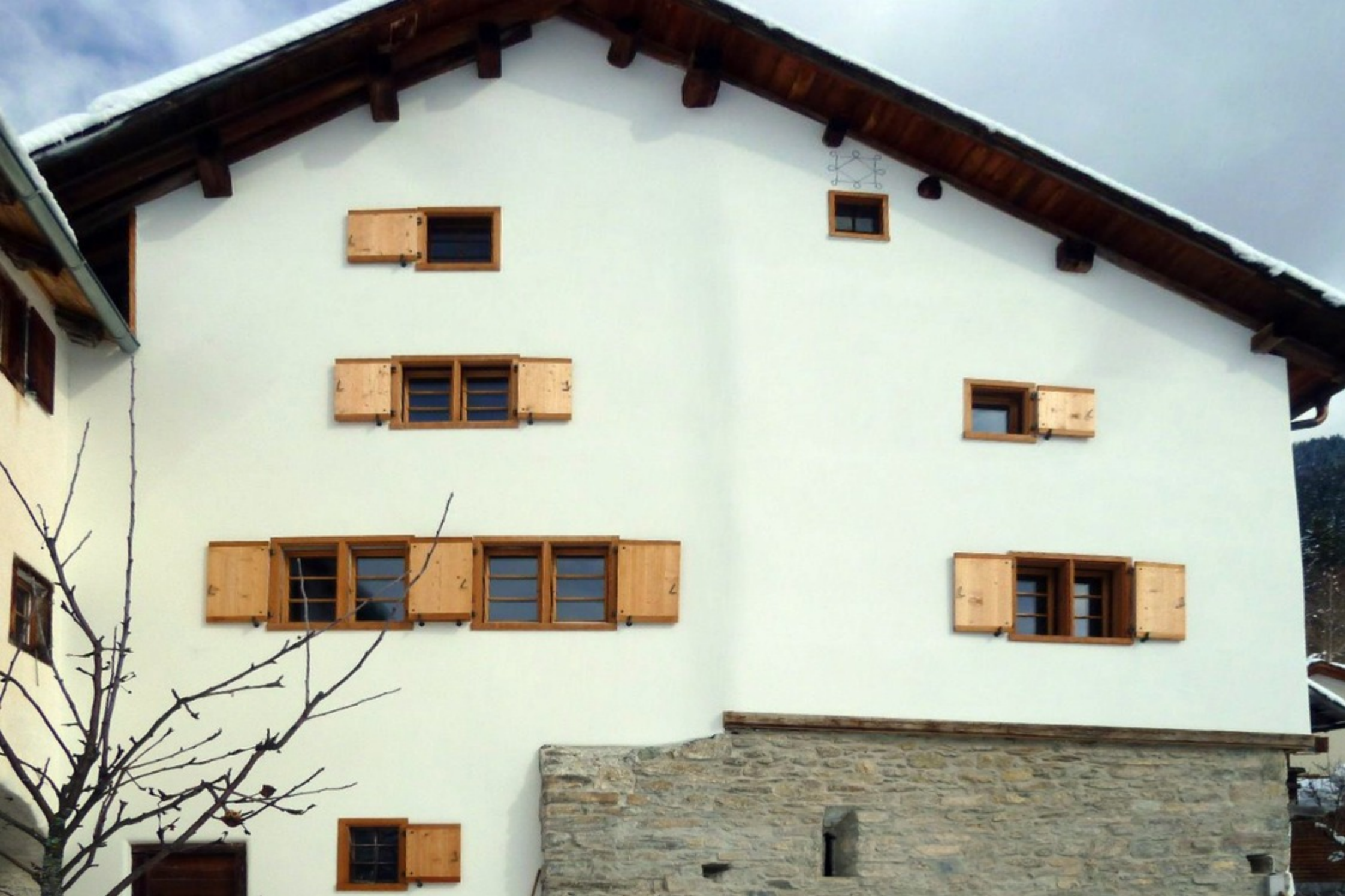
Historic building 'Barandun' Renovation Zillis
