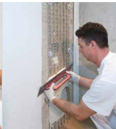
Elaborare (RÖFIX Stucanet) ponte fessure
