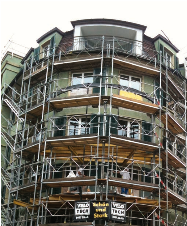
Balkonbau in Zürich Fixit 508 Pump Trockenbeton C30/37
