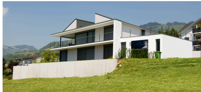
Detached house in the canton of Schwyz, Switzerland
