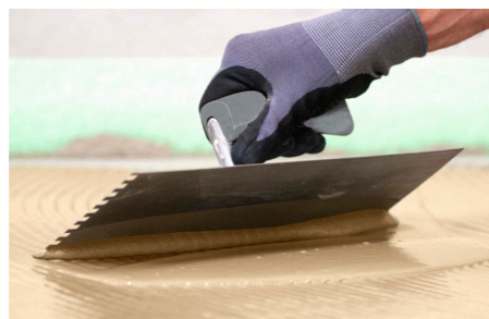
Screed and flooring systems
