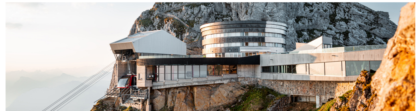
Waiting room extension "Pilatus Kulm mountain station", Switzerland
