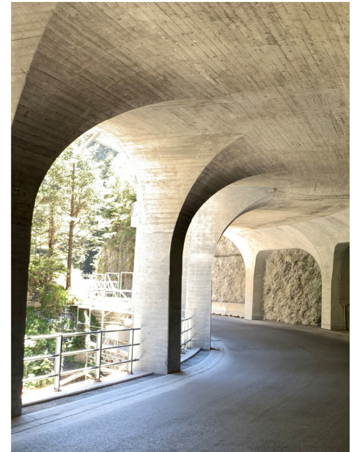
Renovation of the "Viamala 1 gallery", Switzerland
