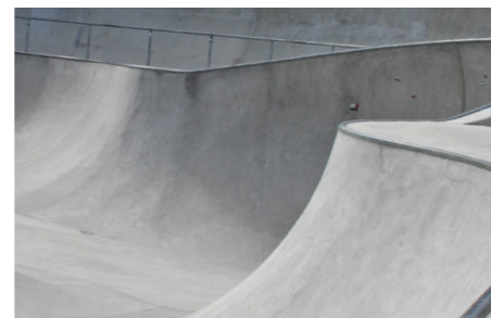
Concrete and civil engineering
