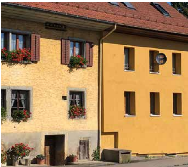
The facade of the building on the right has been newly insulated, but in the process the history of the house has been lost.
