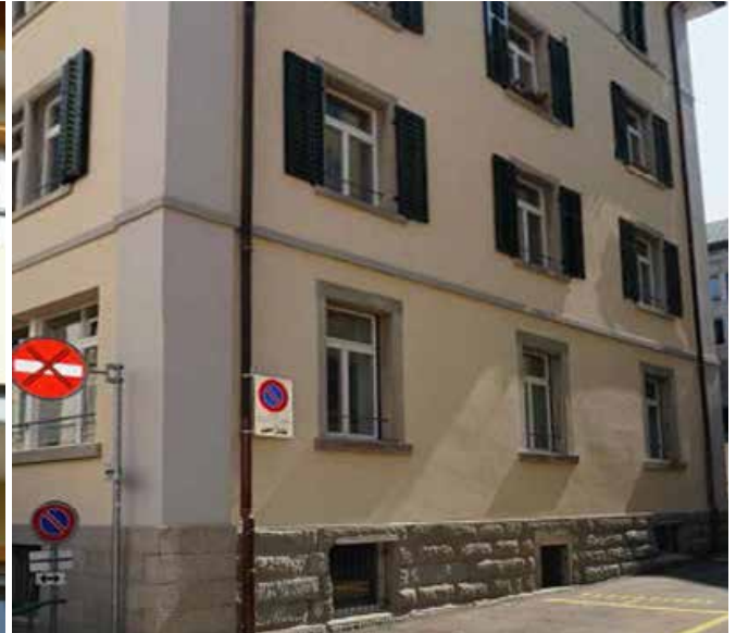
Facade of Aerogel insulating render. The insulation is not visible.
