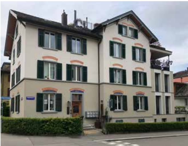
10-year-old Aerogel facade given no maintenance
