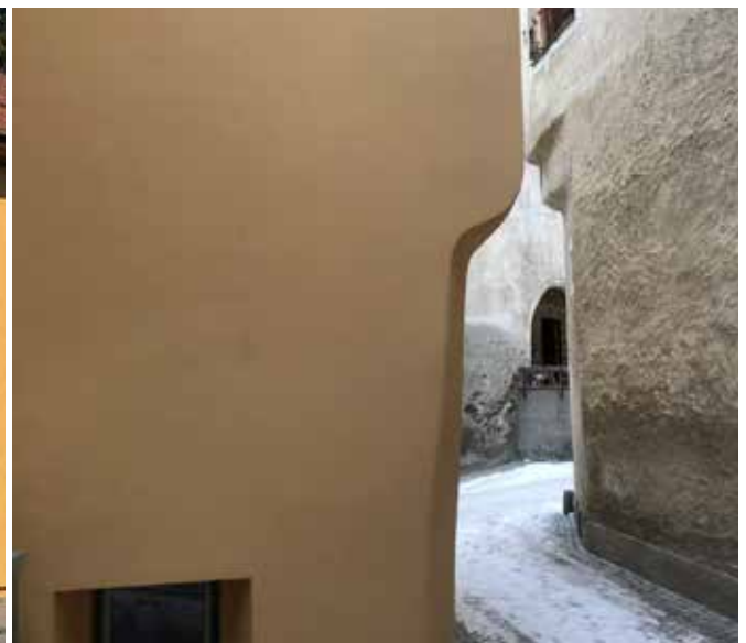
Here the facade created with Aerogel insulating render is telling a story that is still understandable in its context.
