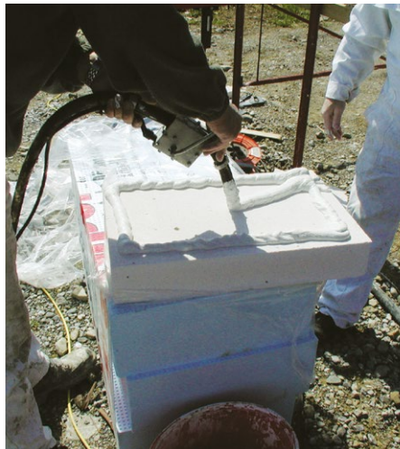
Rand-Wulst-Streifen (maschinell)
