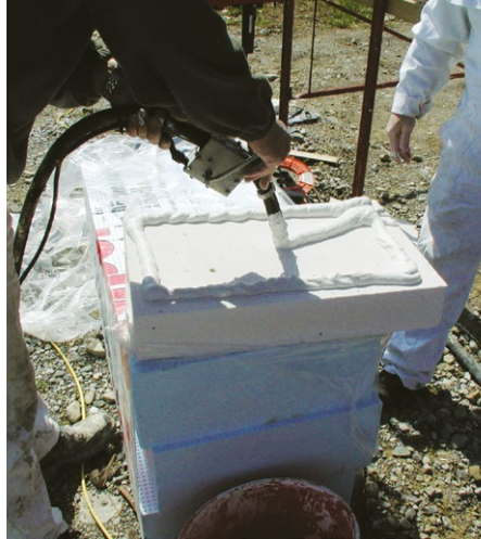
Rand-Wulst-Streifen (maschinell)
