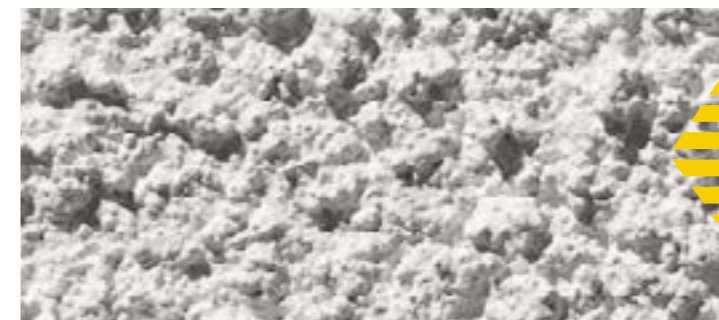
Spray plaster structure
