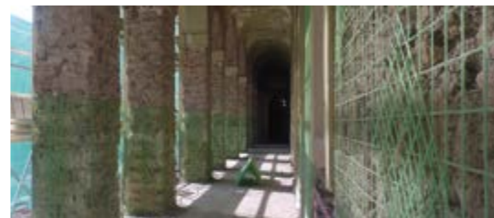
Mechanical strength of the masonry
