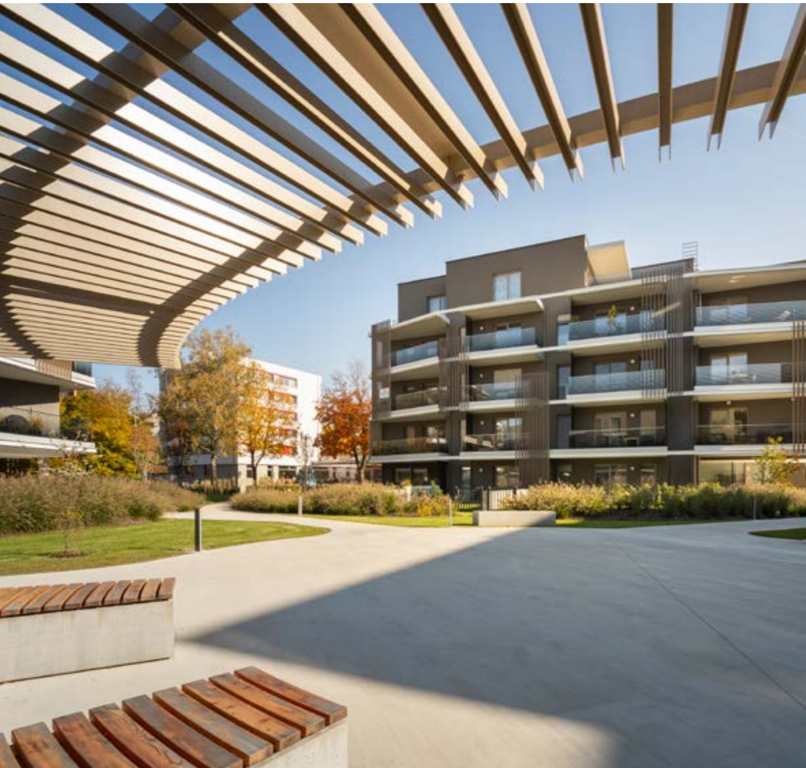
Residential complex "Das Levels", Linz, Austria
