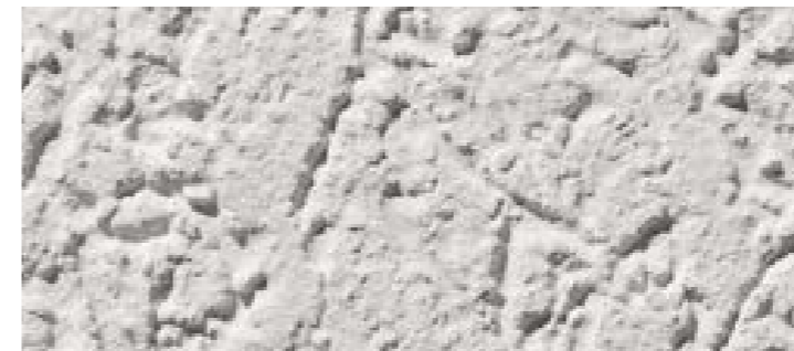
Grooved plaster structure
