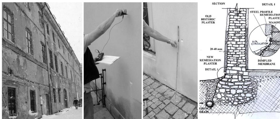
Fig. 1. Southern wing of the castle in Valasske Mezirici not yet renovated in 2007 (left), sampling in northern wing after renovation in 2018 – humidity measurement and height of a sample (middle), typical section and detail (right), source: photos of the author.
