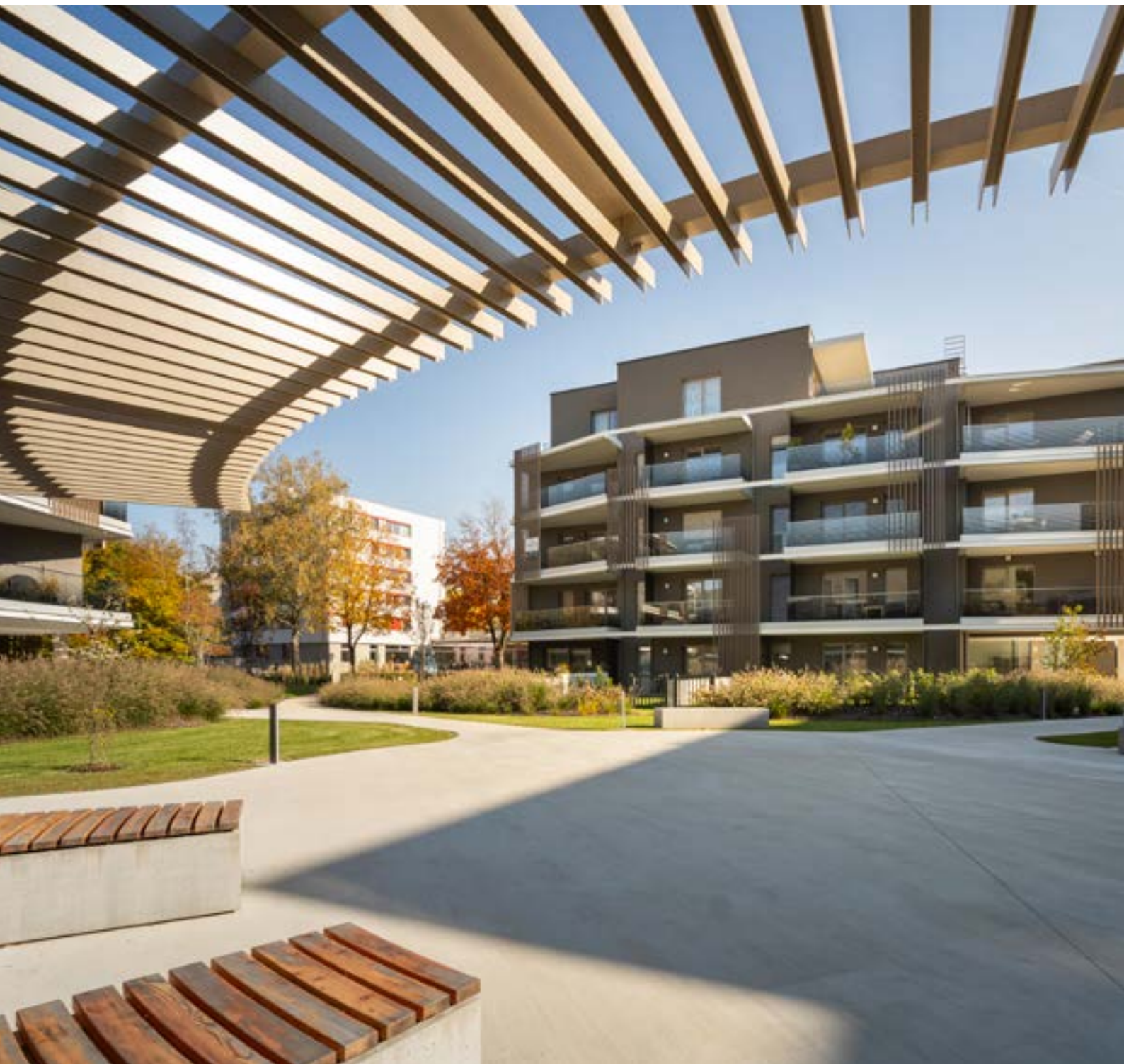
Residential complex "Das Levels", Linz, Austria
