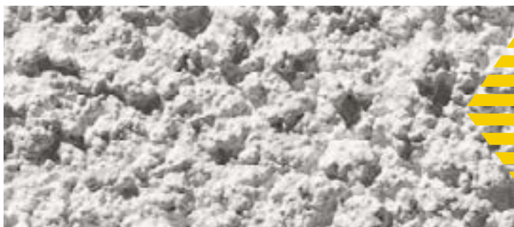
Spray plaster structure
