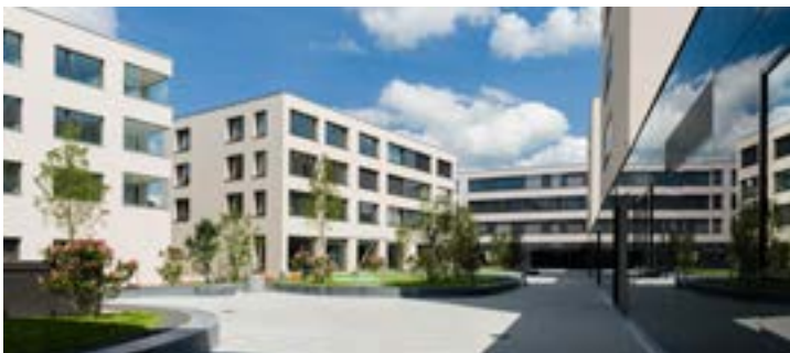
Residential and commercial building, Baar
