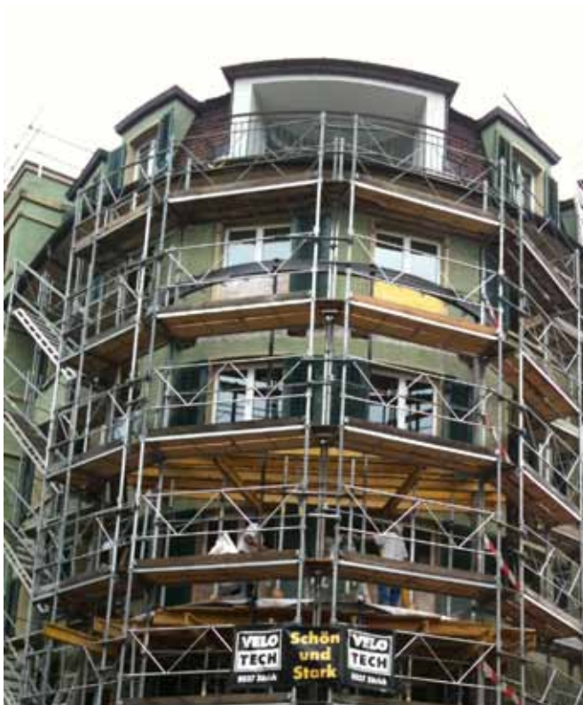
Balkonbau in Zürich Fixit 508 Pump Trockenbeton C30/37
